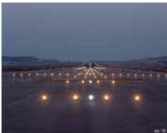
Flexible Pavements in Airfield & Roads Athens International Airport El. Venizelos
