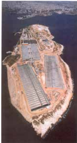
Sewage Treatment Plant of Athens & Peiraeus Psyttaleia
